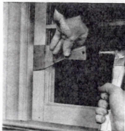
Tapping with stiff putty knife between molding will break the seal
