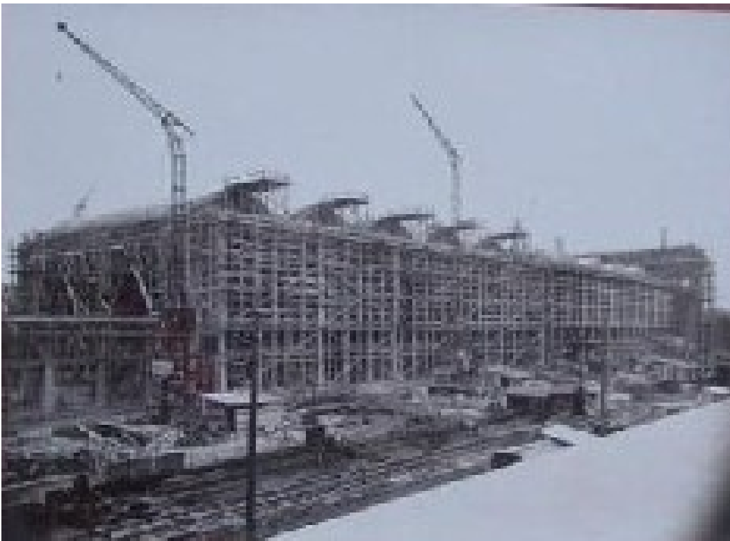
Photographs from a 1928-1929 scrapbook of Dyckerhoff & Widman projects. This appears to be the Frankfurt Grossmarkthalle under construction. Private collection.
