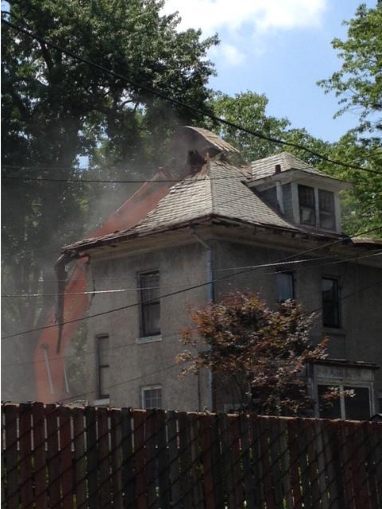
Demolition of 3823 Morrison Street, NW, June 17, 2014
