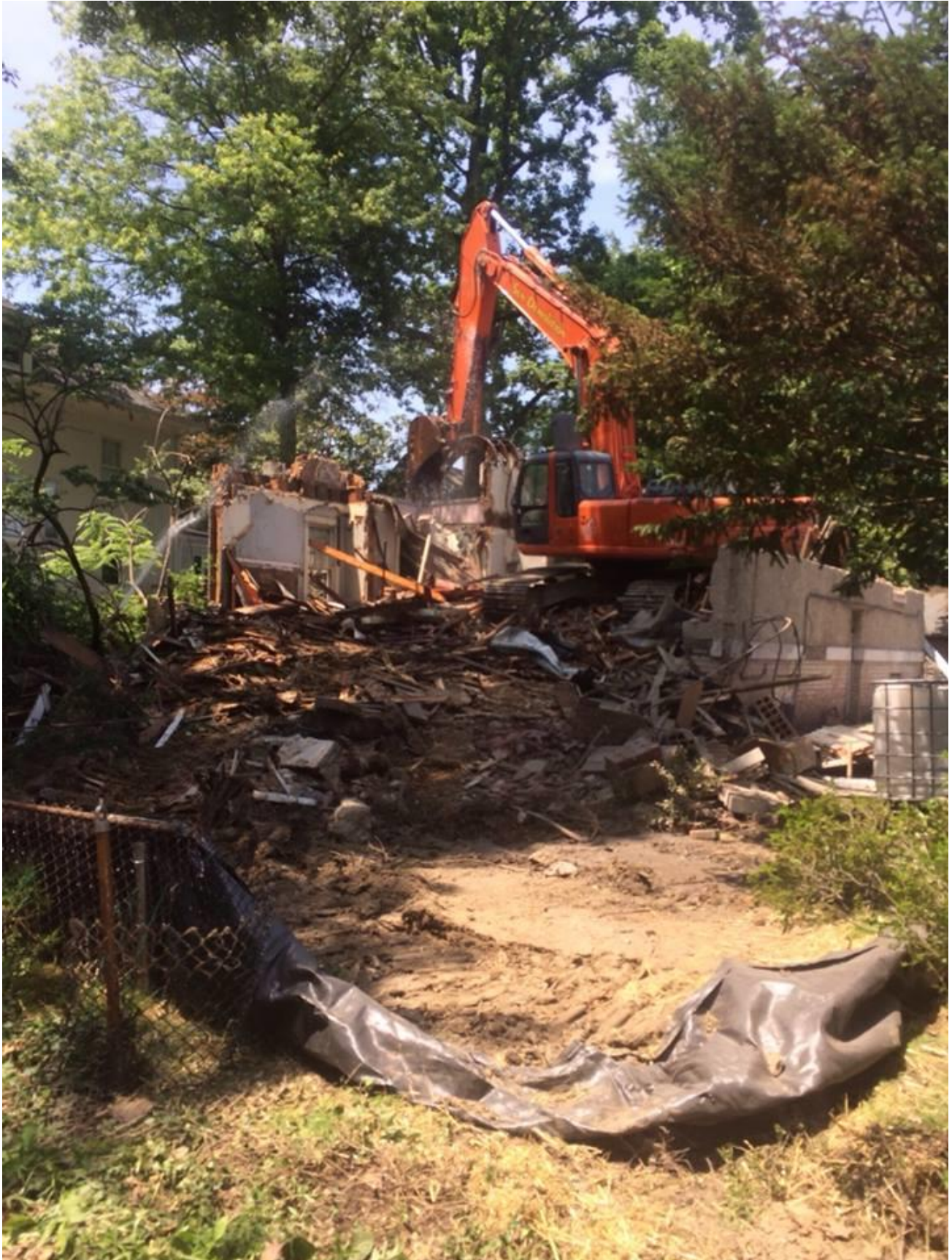
Demolition of 3823 Morrison Street, NW, June 17, 2014
